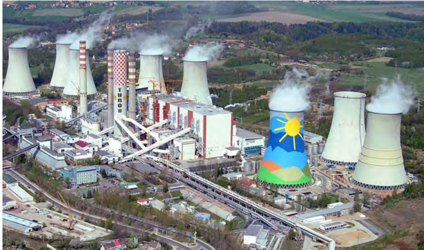
Example of repowered power plant: FB boilers in Turow (Bogatynia), Poland
